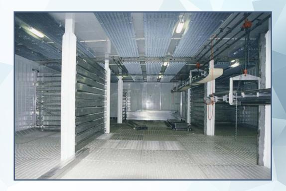
The air coolers are designed for mounting below the deckhead and operates by means of gravity (natural) air circulation.
